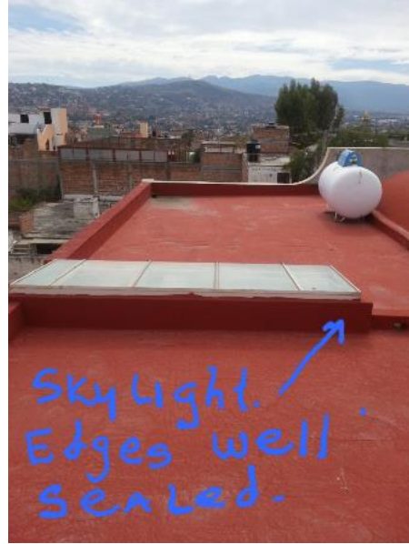
Perimeter of tilted skylight well sealed,
