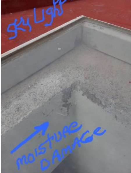
Condensate in bath below collects on glass & drips
